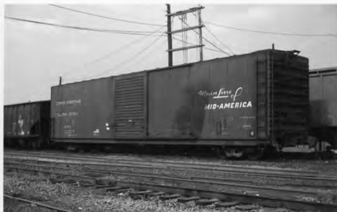
IC 43874. 60FT SD BOXCAR. 43800-43906. Thrall 1965. 70 ton capacity.
